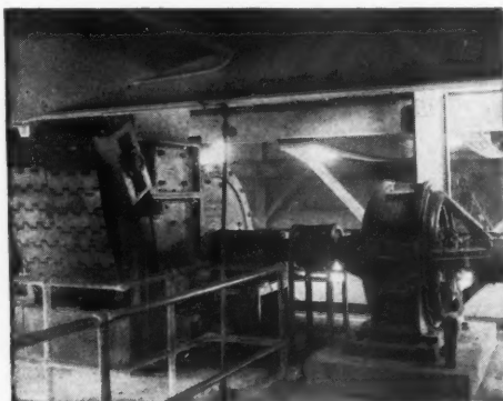
A Hammer Mill in Cement Plant
